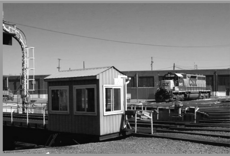
A CSX SD40-2 rests on a roundhouse lead track leading from the steam era turntable at CSX's Cumberland Shop complex. Part of the roundhouse is used by GE to maintain the GE locomotives assigned to the Cumberland Division.
